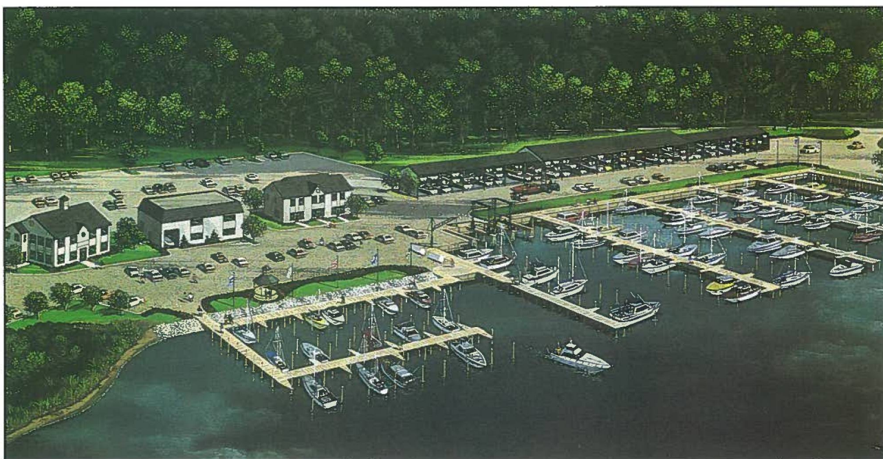
Marinas provide a sheltered harbor for yachts and small boats. Piers extend into the water and finger piers project from them. Each boat's space is called a slip. A self-propelled sling lift ( center ) hauls boats out of the water and a gin pole helps with unstepping masts. Powerboats less than about 25 feet (7.6 m) long are often stacked in dry storage ( background ) with a large forklift truck. They are taken off the rack and launched for each outing.
